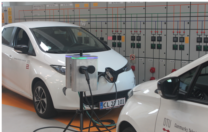
Figure 3. Experimental setup implemented: The figure shows the two Renault Zoes and the charger used in the test. The test is conducted in the DTU Energy System Integration Lab (SYSLAB).
