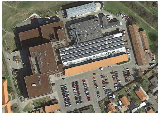
Figure 2 – Top view of the campus (photo taken from Google earth)
